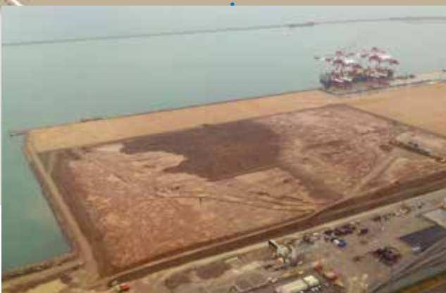
MOVEMENT OF PRE-LOADED MATERIALS (ACTION 6) PRAT TERMINAL
