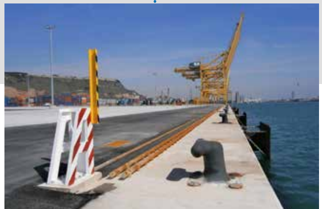
ENLARGING THE MANOEUVRING AREA ON THE SUD WHARF TERMINAL
