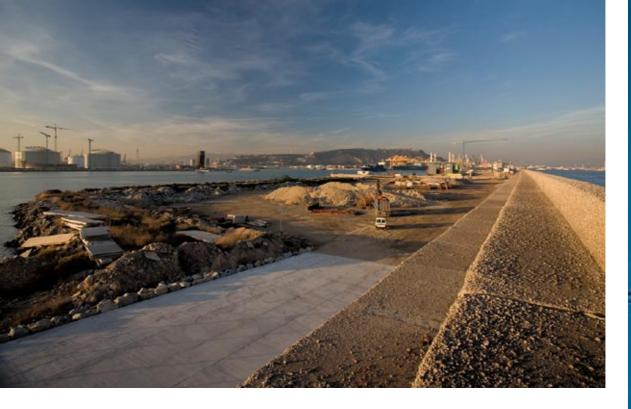
The increasing trade in liquid bulk in the Port of Barcelona and the forecast future demand for handling such goods were the reason for building a new berthing point for this type of traffic. The project called **Berth for liquid bulk carriers** involves building a berthing area for the transfer of refined products between ships and land on the northwest face of the Inflammables wharf.
